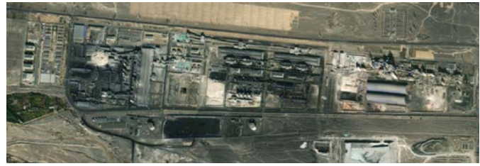
Xinjiang Mahatma complex in Alehui Town, Toksun (Tuokexun) County. 53 Coordinates: 42.824936730621, 87.91506344380534
