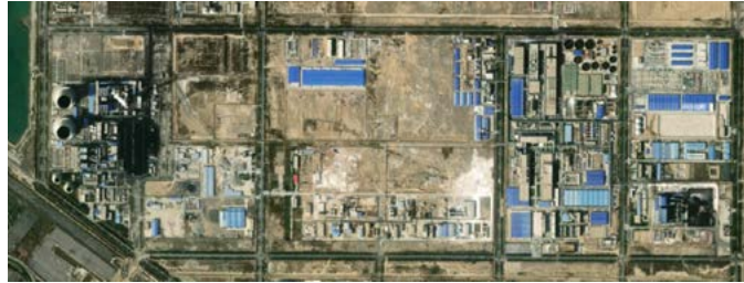
Xinjiang Qingsong Building Materials complex, including Aral Qingsong, near Aral city. 134 Coordinates: 40.592904, 81.197462.
